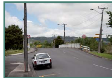
Rail over bridge Waihoehoe Road
