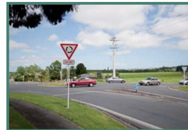
Mill Road roundabout
